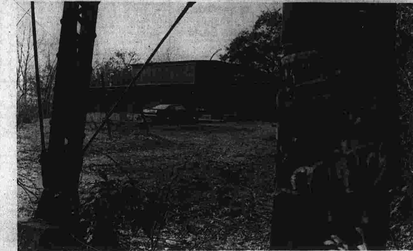
This is the filter plant located off Cooper Hill St.
